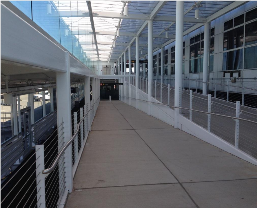
C10 Walkway & Adjacent AAG Walkway
